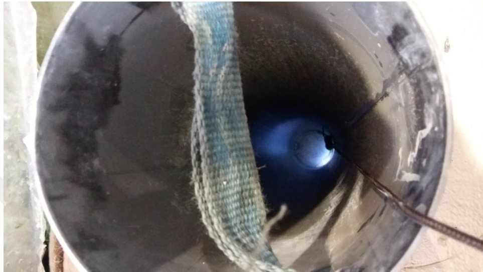
Figure 4.13. Photograph depicting the inside of the driven casing pipe illuminated with a suspended torch.
