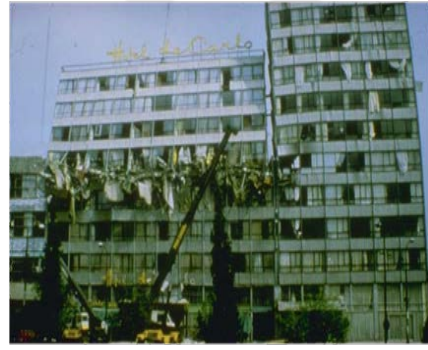
1985 Mexico City depremi hasarı [Arnold, 1989]
