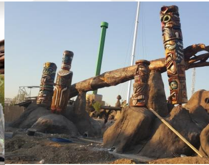
Figure 4.68: Rocksfear Entrance (Photograph by G. Eyüboğlu)
