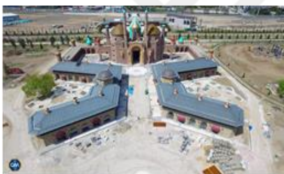
Figure 4.13: Ankapark Entrance Complex from the inside 390
