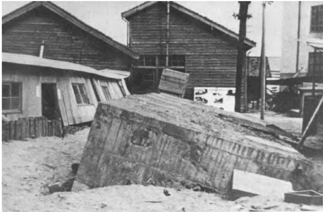
Figure 1.3 : Floating of a buried tank after Niigata (Japan) earthquake in 1964 [3].
