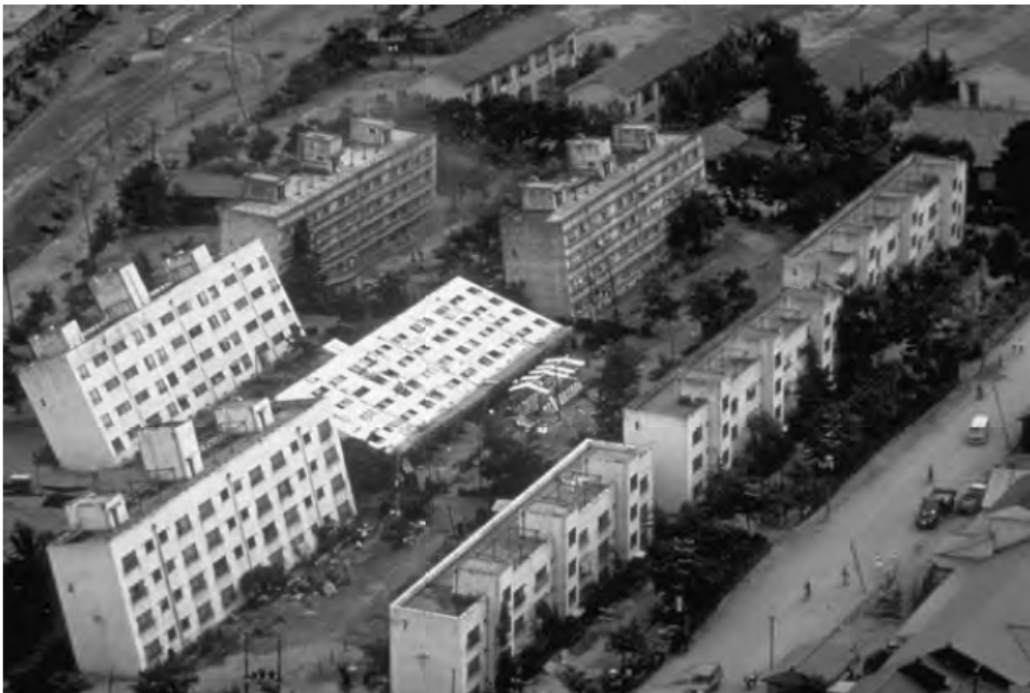
Figure 1.2 : Tilting of apartment buildings after Niigata (Japan) earthquake in 1964 [3].
