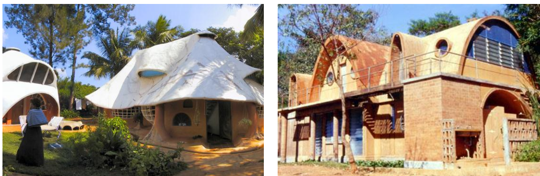
Figure 4. 4 : Architectural styles and materials of Auroville ( https://www.auroville.org ).
