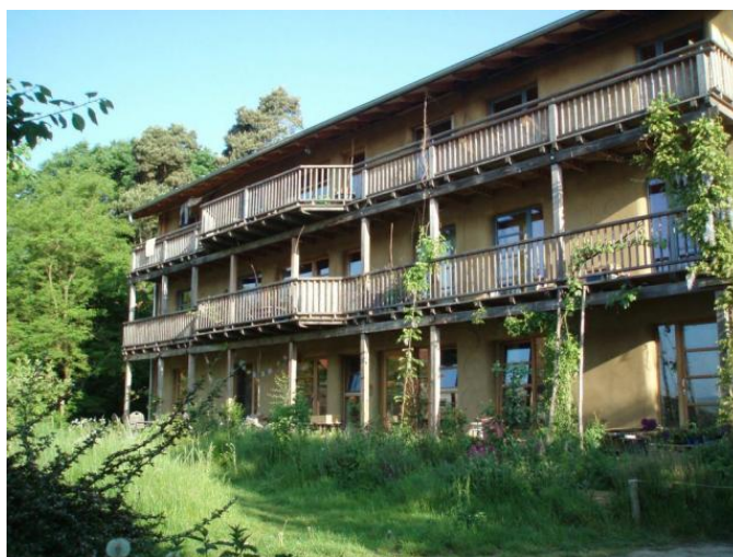
Figure 4. 22 : The 'Strohpolis' house in the ecovillage of Sieben Linden - Europe's largest house made out of bales of straw ( http://www.environmentandsociety.org ).
