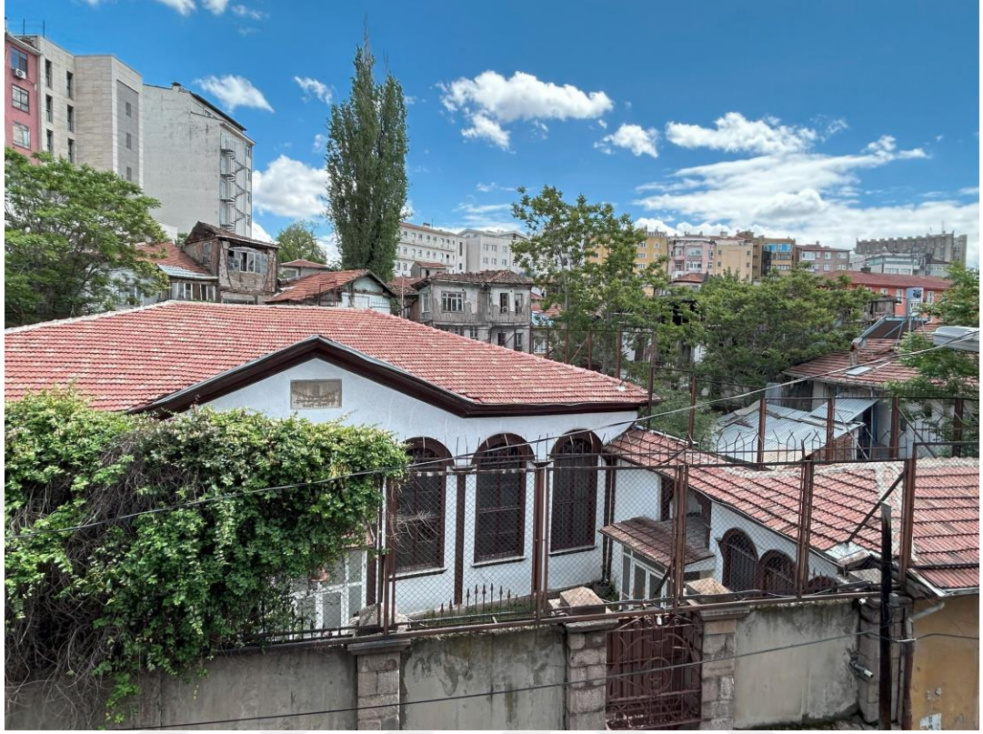
Figure 3.62. Ankara Synagogue, Courtyard and Walls (Author, 2024)
