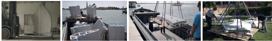
Şekil 4. 18 Blokların nakliyesi (Block Research group, 2021b; Block Research group, 2021c)
