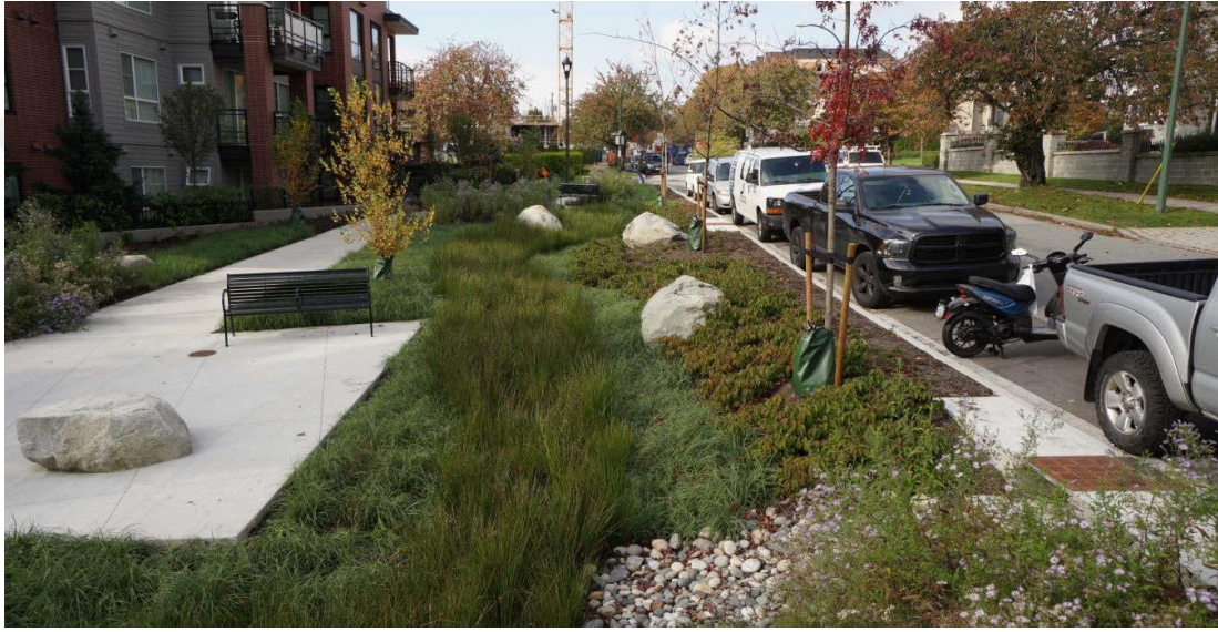
Şekil 2. 24 Vancouver'ın Yukon Sokağında ve 63. Caddesinde biyolojik hendek kurulumu. Kaynak: Conger, T., Couillard, A., Hoog, W., Despins, C., Douglas, T., Gram, Y., Javison, J., Lukes, R., Owen, C., Pollard, M., Satzewich, J. ve Scholefield, M. (2019). Rain City Strategy . City of Vancouver. https://vancouver.ca/home-property-development/green-rainwater-infrastructure-policies-and-reports.aspx .
