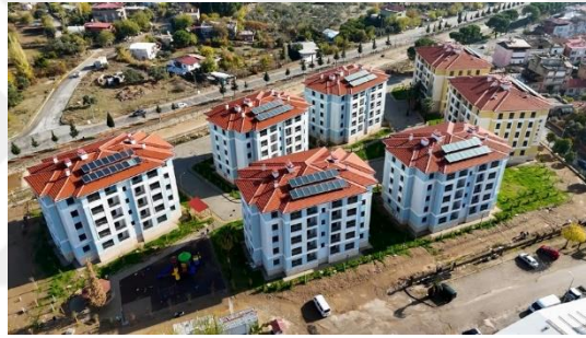
Figure 26. TOKİ Housing Complex in Aydın (Source: Aydın, TOKI)
