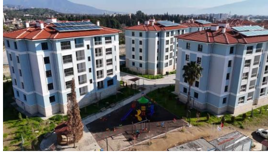
Figure 25. TOKİ Housing Complex in Aydın (Source: Aydın, TOKI)
