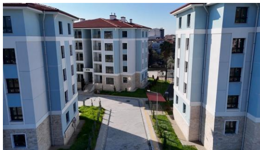
Figure 27. TOKİ Housing Complex in Aydın (Source: Aydın, TOKI)
