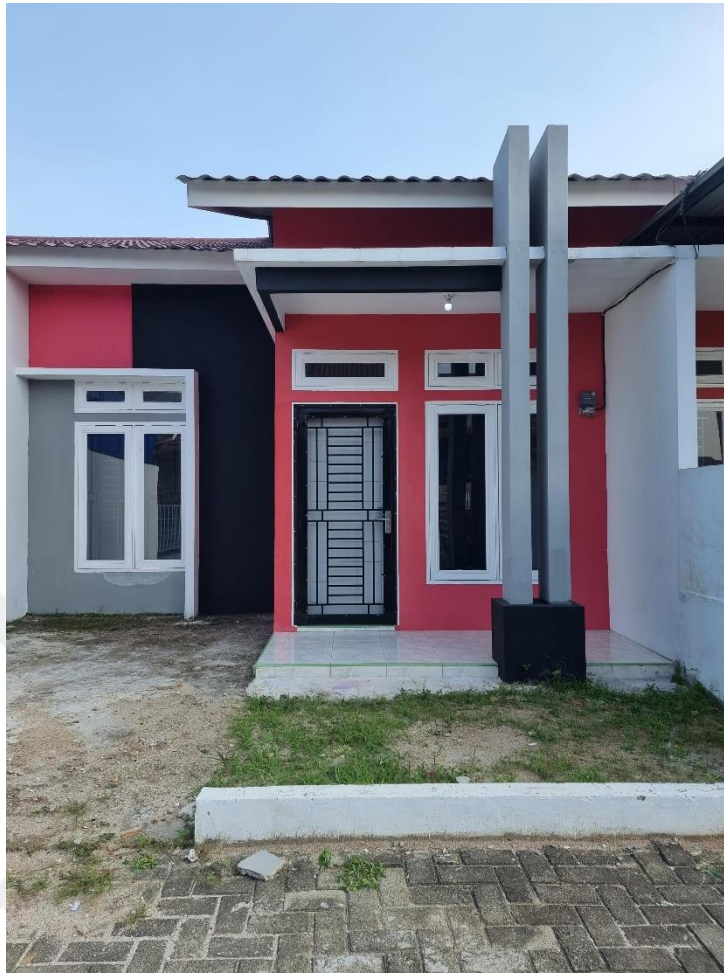
Figure 1.2. One of non-engineered masonry house front view.
