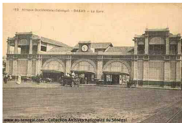
Figure 21: Dakar train station in the past
