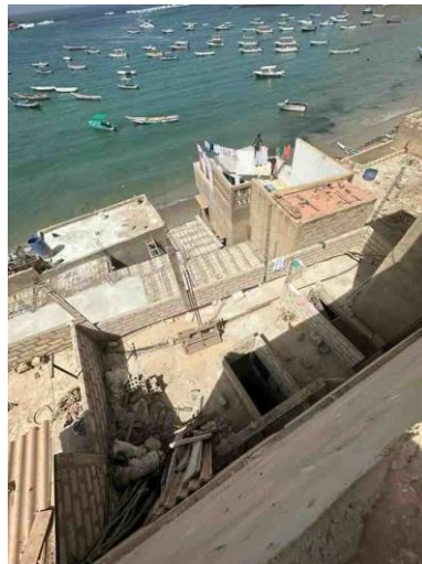
Figure 139: Expansion (ID_13) of Traditional House for More Space (Author)
