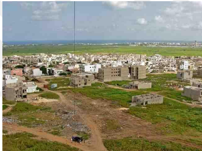
Figure 49: Buildings under construction in Yoff (Dakar, Senegal)
