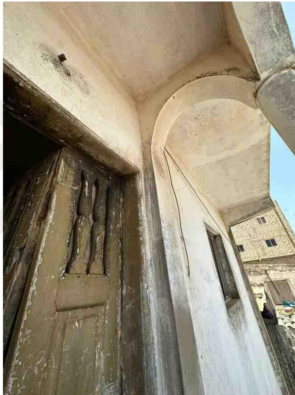
Figure 104: Ornamentation of a traditional house which has undergone modifications (Author)
