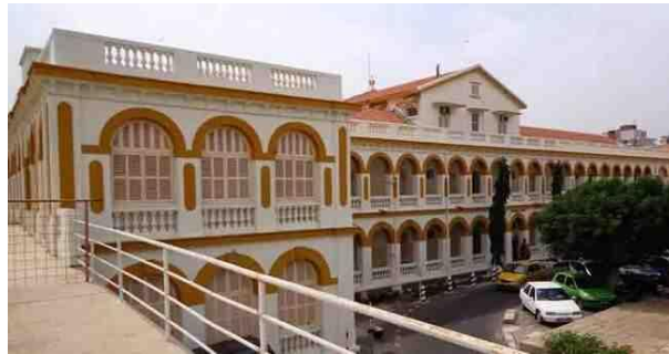
Figure 53: Dakar Main Hospital
