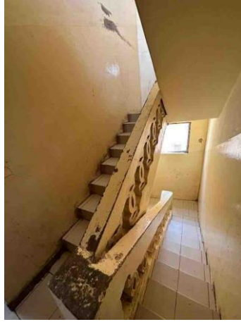
Figure 137: Renovated Traditional House Stairs (ID_10) (Author)
