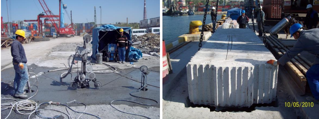
Figure 4-34 Cutting and transporting concrete
