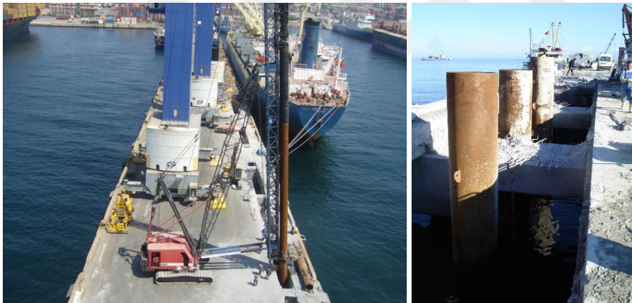
Figure 4-35 Positioning and driving steel pipe piles
