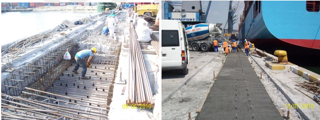
Figure 4-37 Rebar installation and concrete pouring
