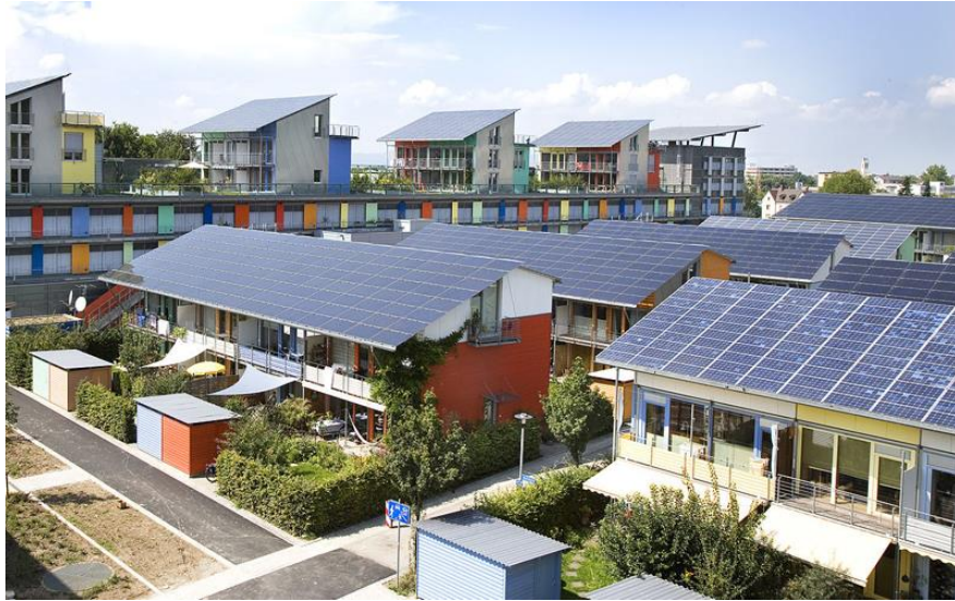
Şekil 8: Fotovoltaik Paneller- The Solar Settlement in Schlierberg, Freiburg, Germany [29]
