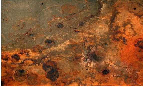
Figure 3 1. Rust the most familiar example of corrosion
