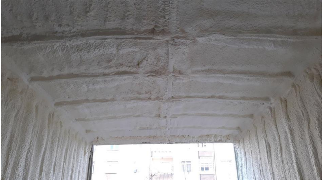
Figure 3.6 Polyurethane Foam Application [30].
