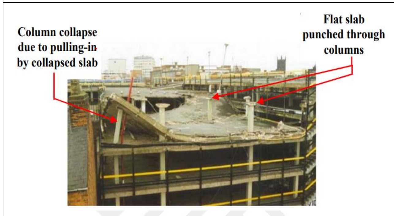
Figure 1.2: Collapse of large area of flat slab due to punching shear
