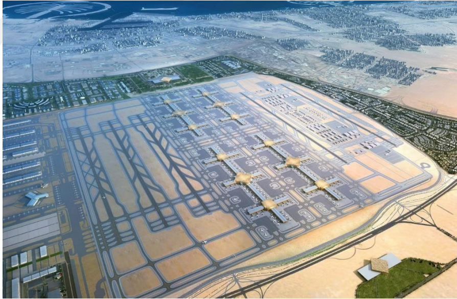
Resim 3. DWC Airport City
