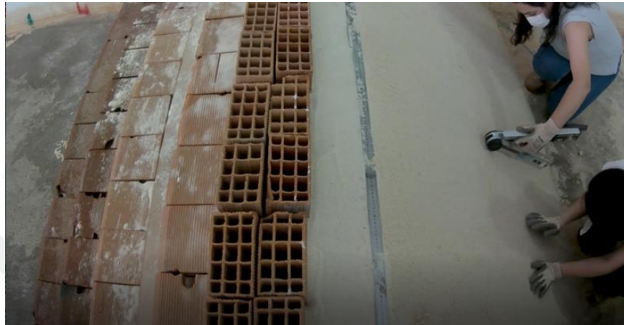
Figure 3. 8: Arrange downstream and upstream slope of dam
