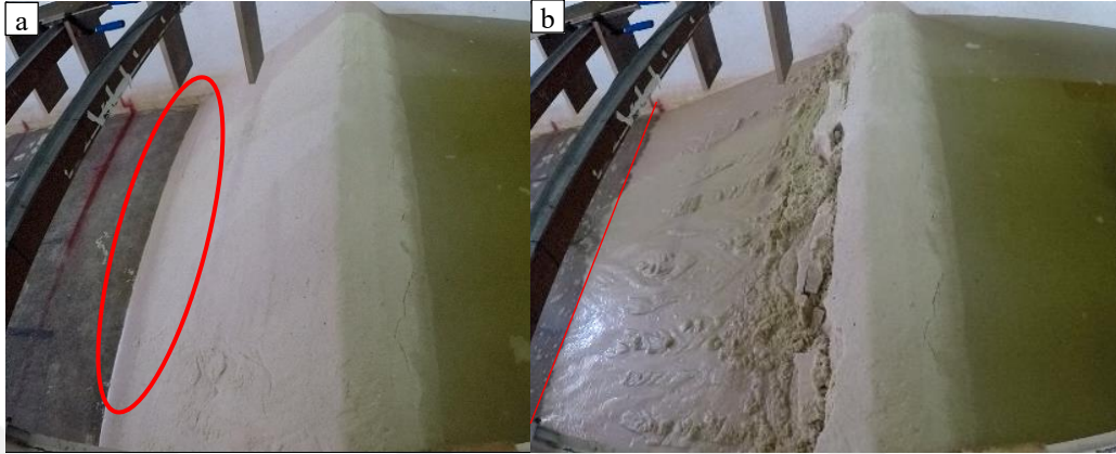
Figure 4.36: Water seepage start from dam body skirt (a) and sediment passing from the red line (b)
