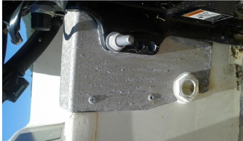
Figure 2.3 Ground to which the engine of a fishing boat is connected.
