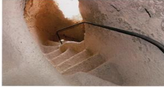
Fig. 14 Eastern Buddha, spiral stair (cont) inside the cliff. For ensuring the visitor's safety a handrail was installed during the rehabilitation measures.
