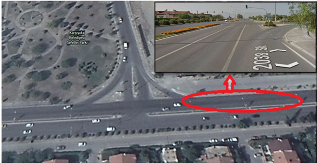
Figure 6.9 Entrance approach where maintenance work will be carried out (Google Earth, 2018)
