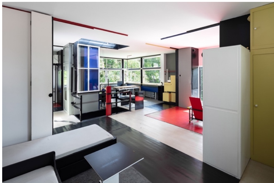
Figure 4.1: Interior view from Schröder House showing sliding partitions
