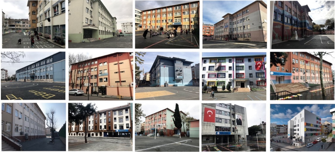
Figure 5.10: Exterior views of the visited school buildings
