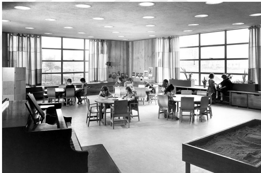
Figure 3.6: Interior view of a classroom at Crow Island School
