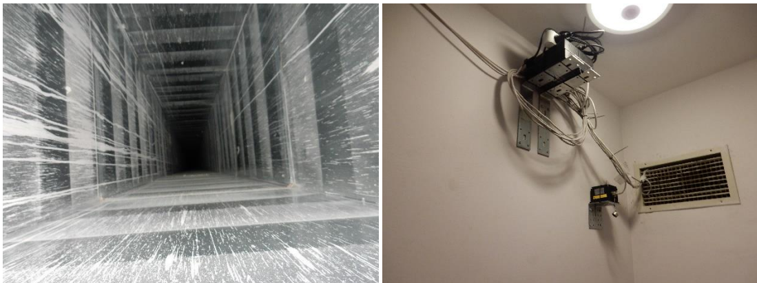
Figure 2.6 : Ventilation shaft and located receiver and the sensor on the 16th floor.
