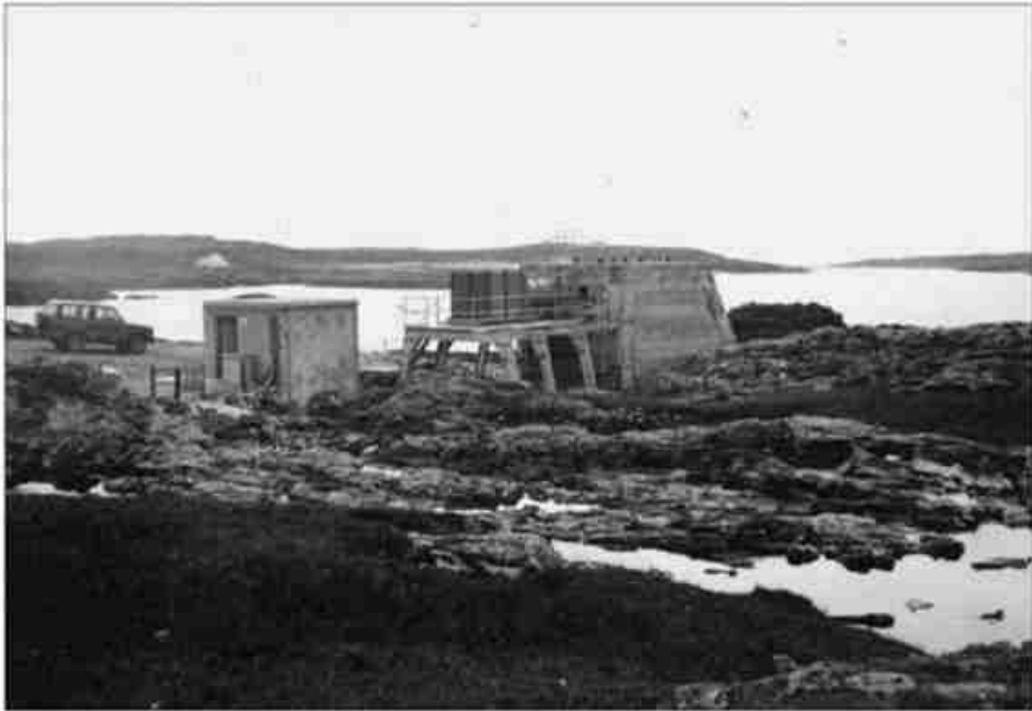
Figure 2-11: The OWC WEC device structure in Islay Project, Whittaker et al. (1997)
