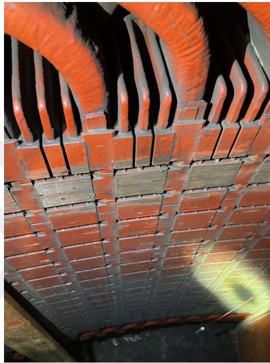
Figure 3.3: Fingers of the Westinghouse generator.
