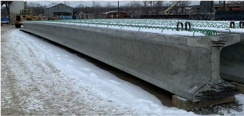
Figure 4.4. 42" x 49" Bulb Tee Beams used in Saginaw Bridge Project
