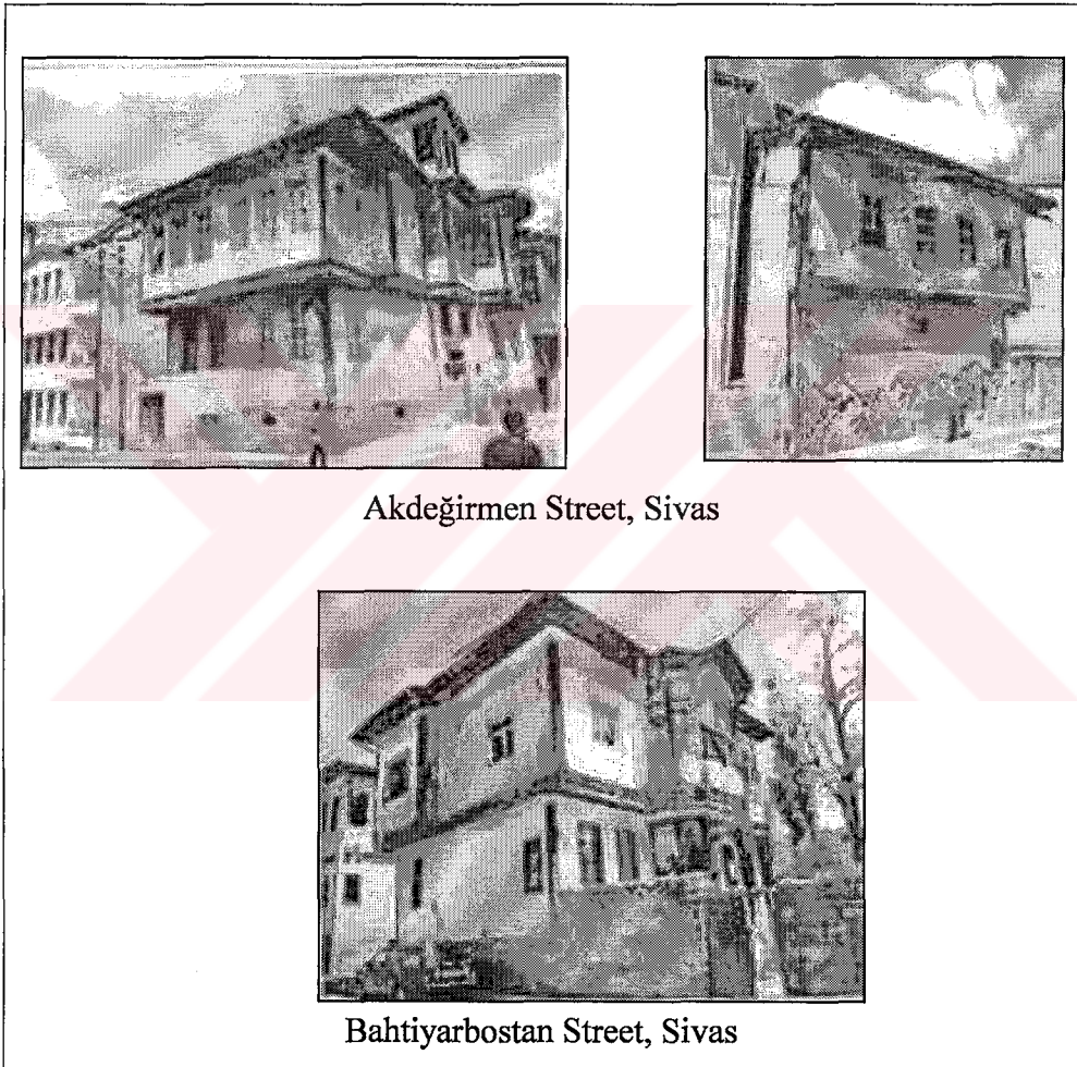
Figure 3.17 Traditional Timber Buildings with Sun-Dried Brick Fill ( http://www.sivas.gov.tr/tarihivasevleri/k14.htm )
