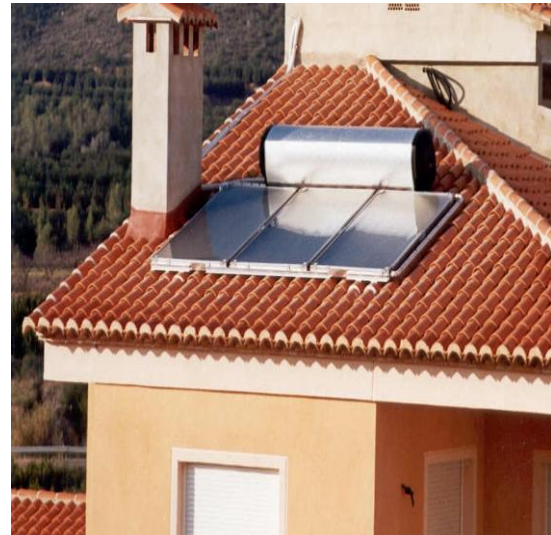
Figure II.13 Thermosyphon System with Horizontal Storage Tank in Gran Canary (ESTIF, 2010)
