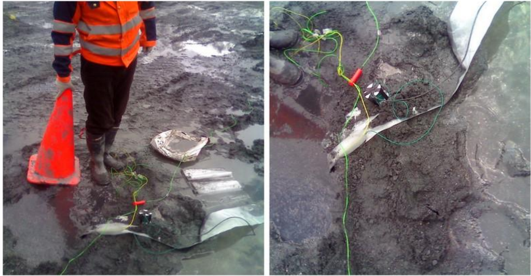
Figure 4.4 Wet hole loaded by bulk ANFO
