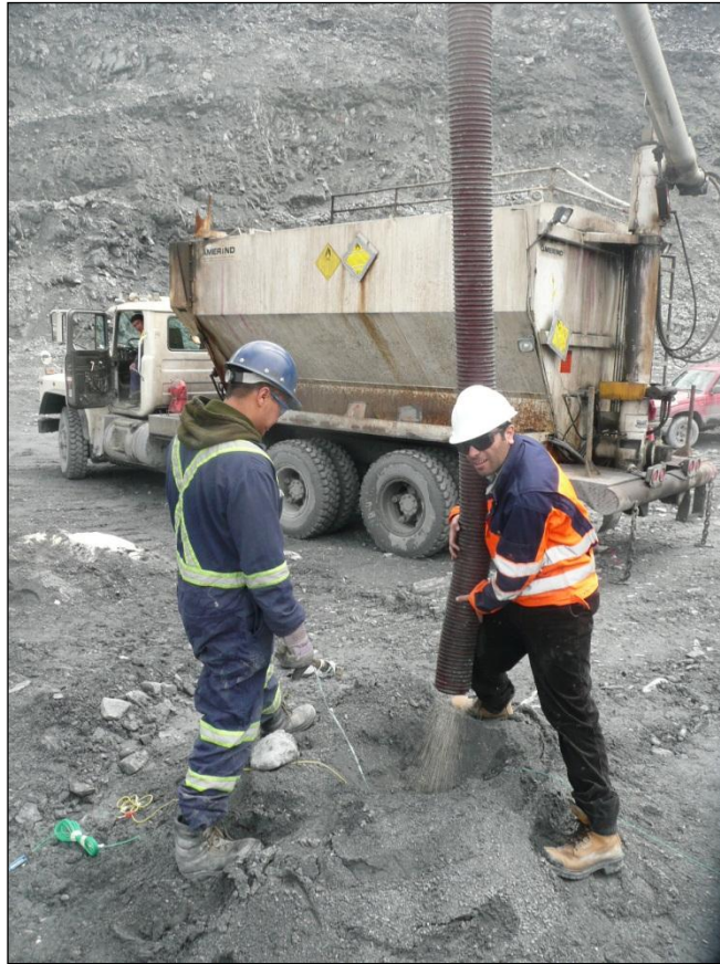
Figure 2.4 Loading blasthole with ANFO bulk truck
