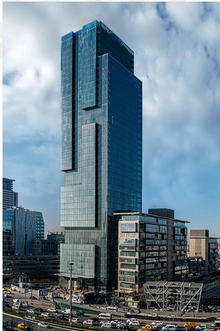
Figure 3.3. General view of the structure.
