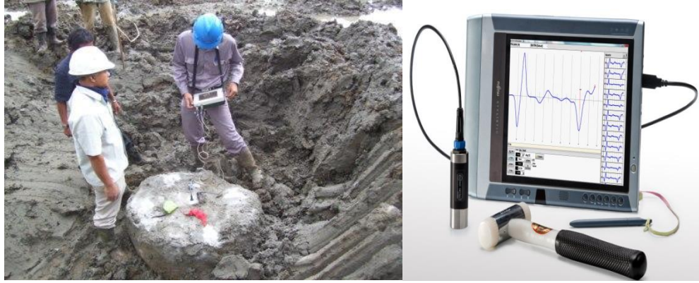
Şekil 3.16. Pile integrity test ( https://diskmal.wordpress.com/tag/loading-test/ )
