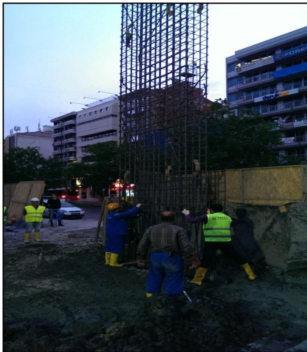
Figure B.4 Placing reinforcement cage
