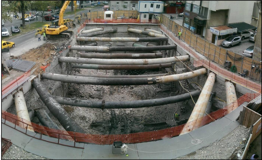
Figure B.7 During excavation stage-1
