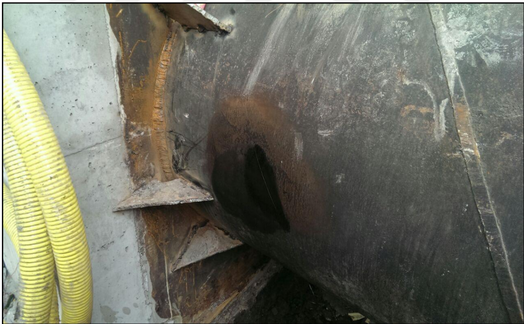
Figure 4.16 Purified bonding area
