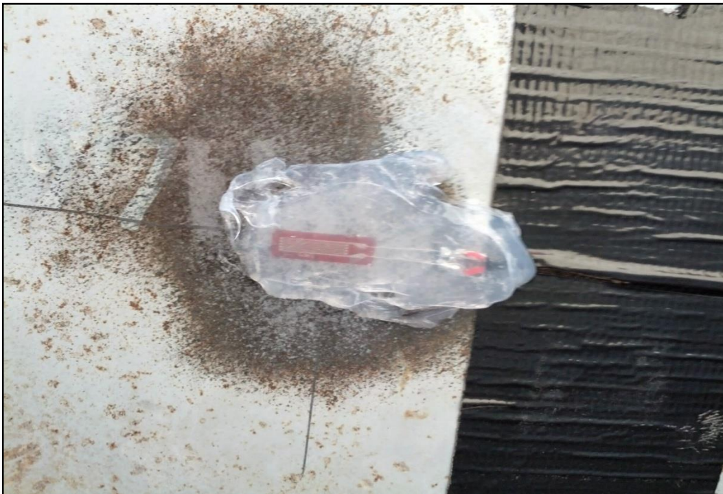
Figure 4.24 Coating the gauge with mastic
