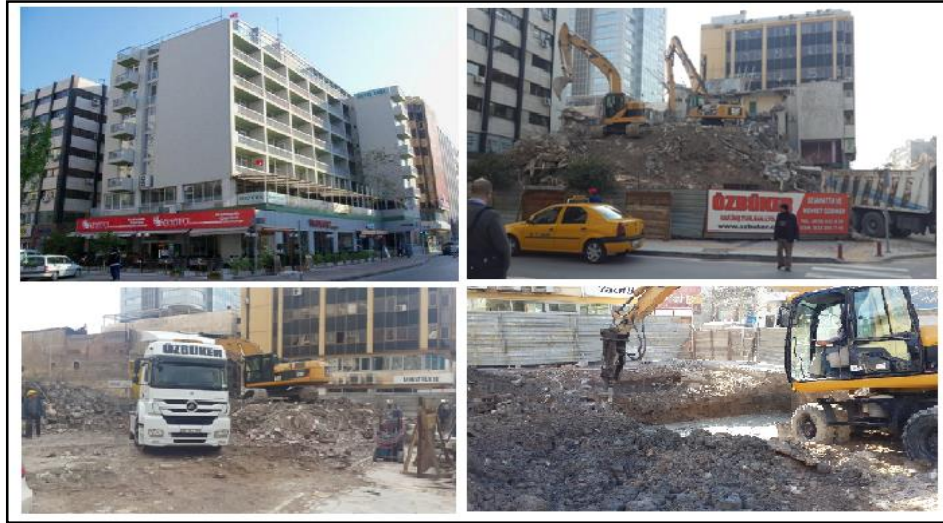
Figure 3.2 Existing building, Anba Otel and its demolition
