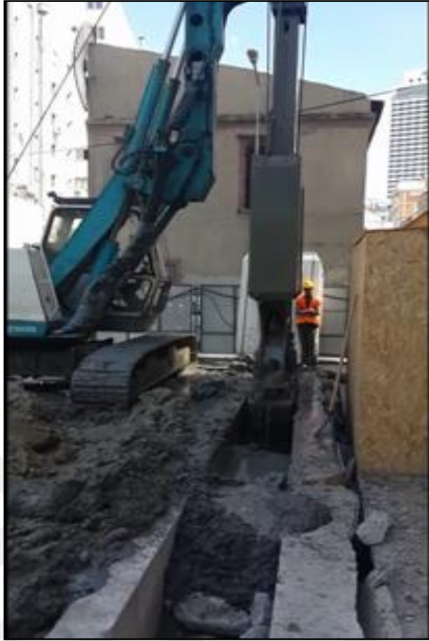
Figure B.3 Trench excavation
