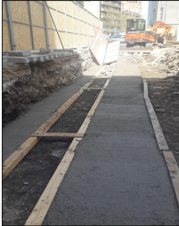
Figure B.1 Preparing the guide wall
