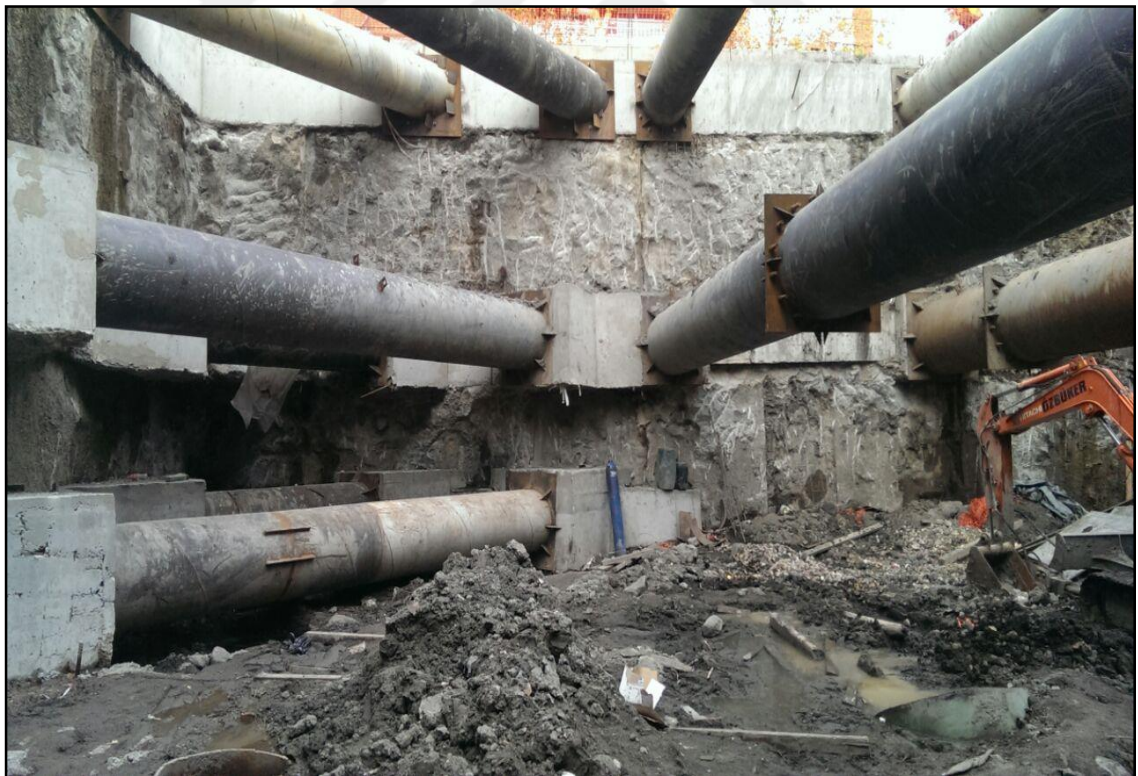
Figure B.8 During excavation stage-2
