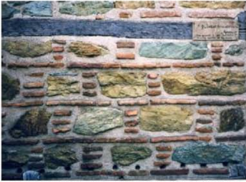
II.1.1.c Cloisonné with horizontal bricks in the joints, at H. Nikolaos Orphanos, Thessaloniki
