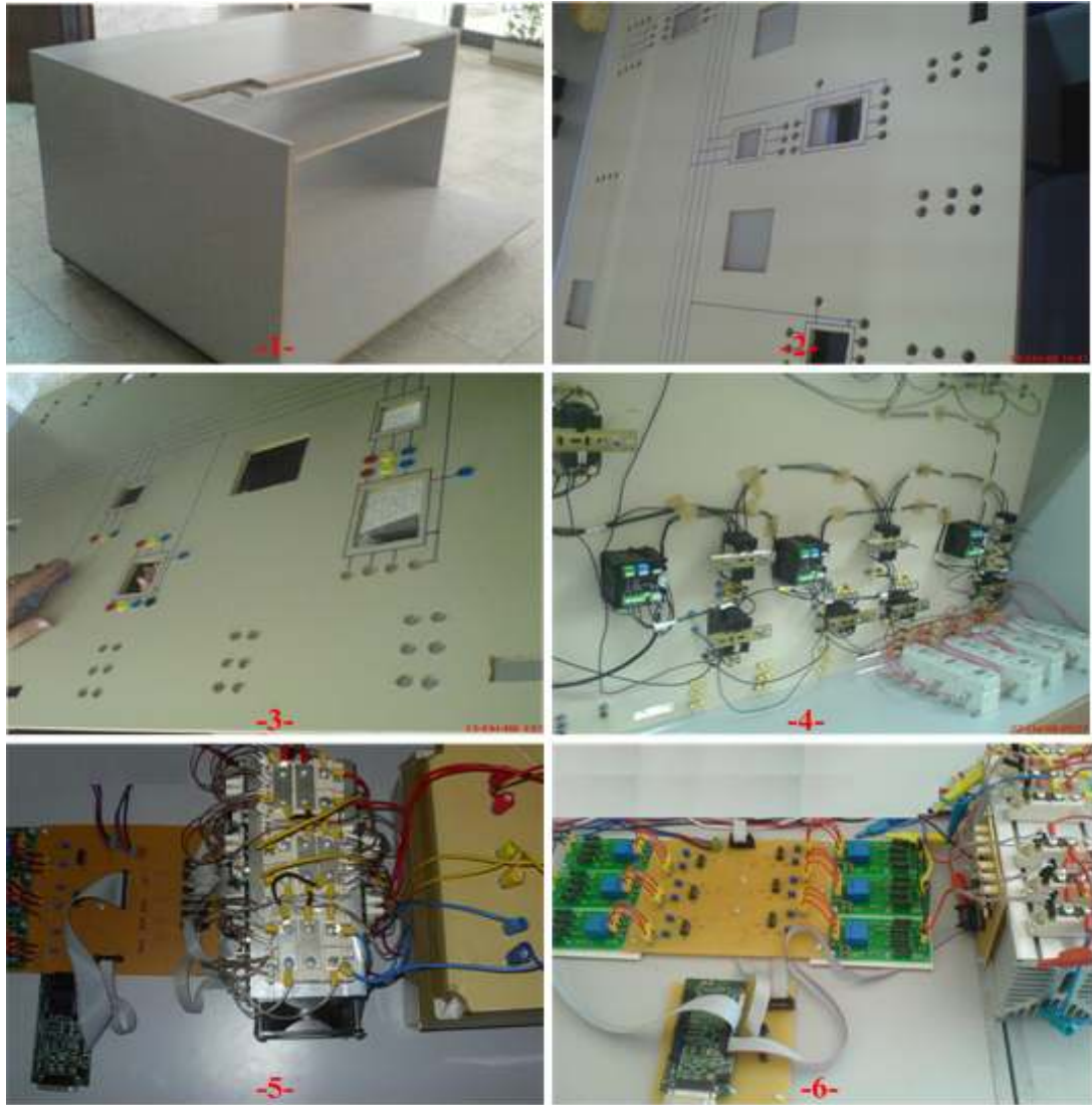
Figure 6.15. The construction stages for the experimental panel of the CPP
