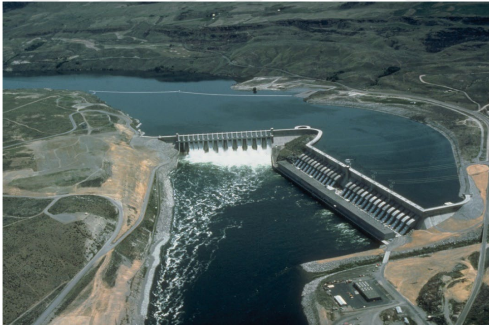
Figure 2.3 Run-of-River Scheme HEPP- Chief Joseph Dam, US [36]
