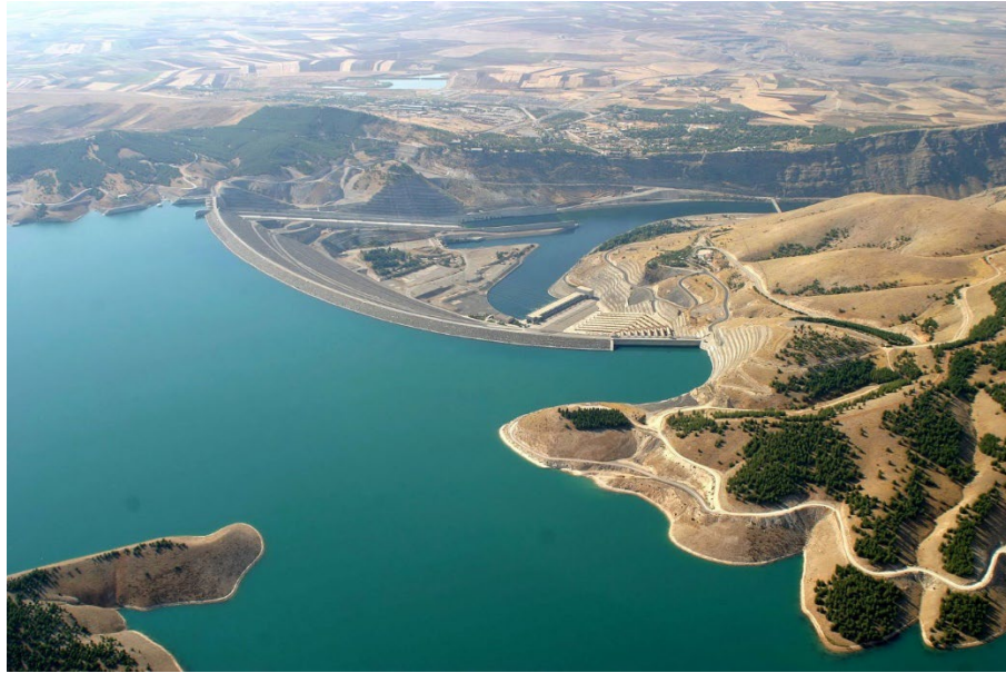
Figure 2.5 Storage Scheme HEPP- Ataturk Dam, Turkey [38]
