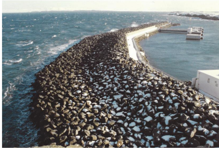
Figure 2.8 Berm breakwater at Helguvik, Iceland (Van der Meer and Sigurdarson 2016)
