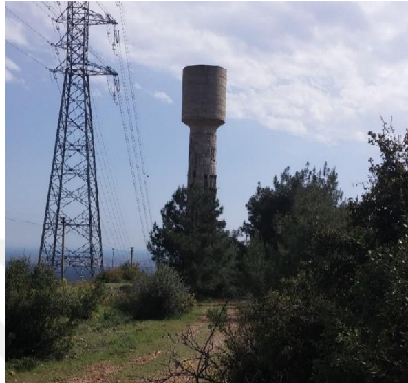
Figure 5.2 Surge Tank of Kepez – I HPP
