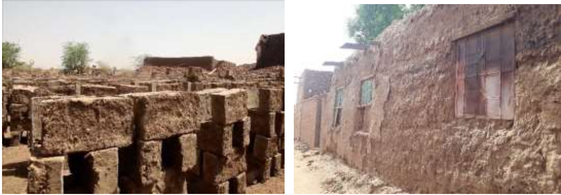
Figure 5.33 The use of clay in the houses
