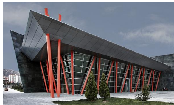
Figure 2.36: Full height glass curtain walls providing views to the outside [54]
