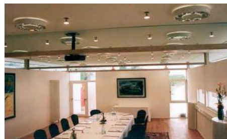
Figure 2.55: Timber-glass composite beams in the conference room in the Palafitte hotel [42]
