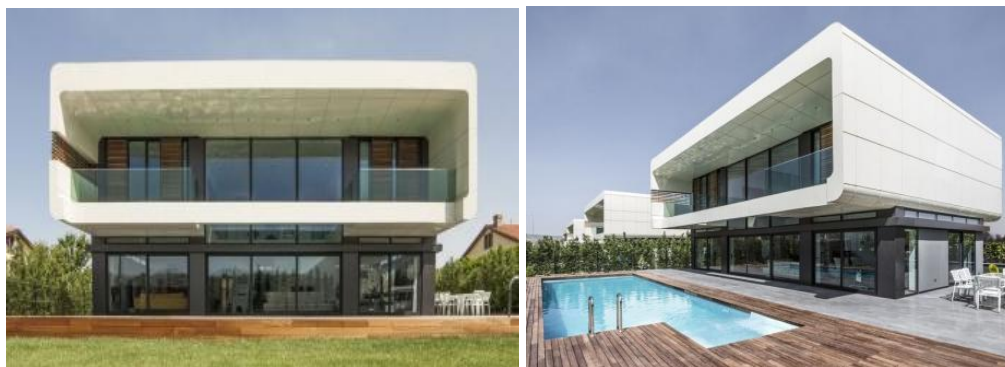
Figure 2.32: Modern home in Turkey [50]
