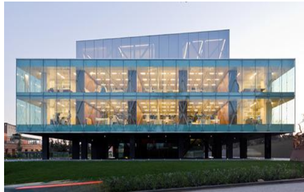
Figure 2.35: Vakko Headquarters and Power Media Center [53]
