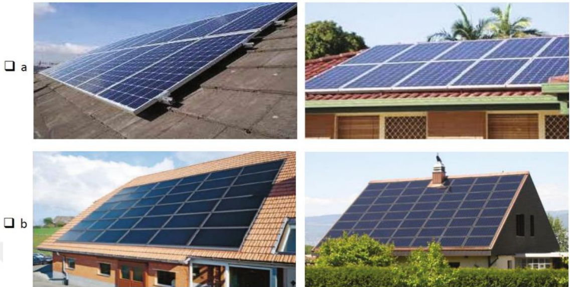
Fig. A.2. Differences between BIPV and BAPV systems.
