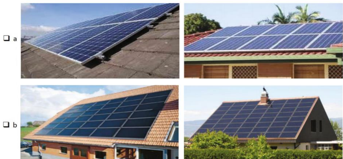
Figure 3.2 Images for Question 20; Differences between BIPV and BAPV system (Joseph, B., Pogrebnaya, T., Kichonge, B., 2019).
