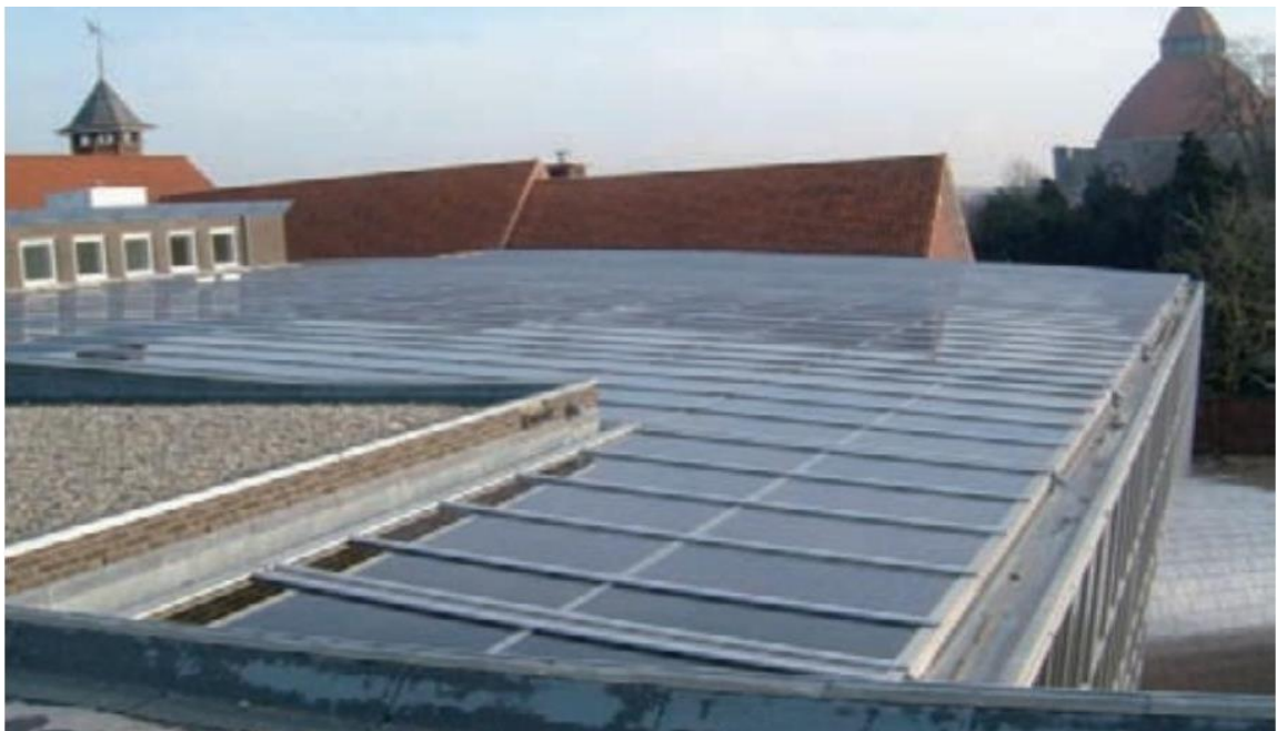
Figure 2.13. The image of Flat Roof in Dongen Town Hall, Germany (Source: URL 7).
