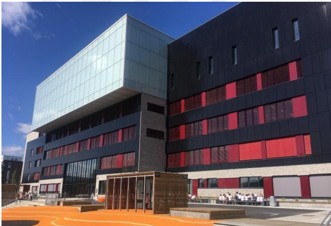
Figure 2.12. The image of Curtain Wall Facade in Brynseng Primary School, Oslo, Norway (Source: URL 6).
