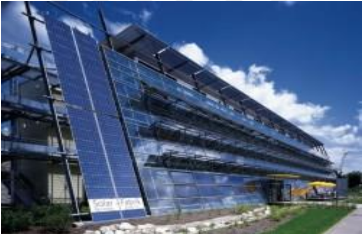
Figure 2.8. Image of a structure with a sunshades/shading BIPV façade (Sheelamkhare, 2013).
