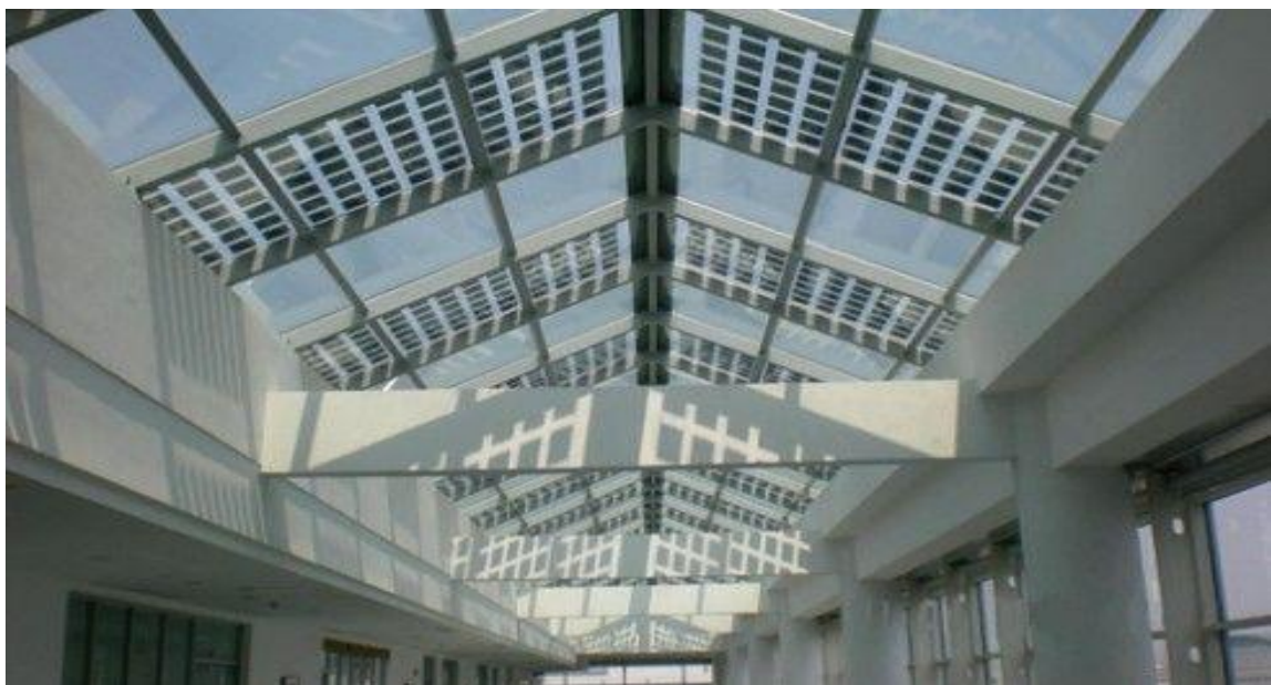
Figure 2.4. Atrium BIPV system application (Djibo, 2018).
