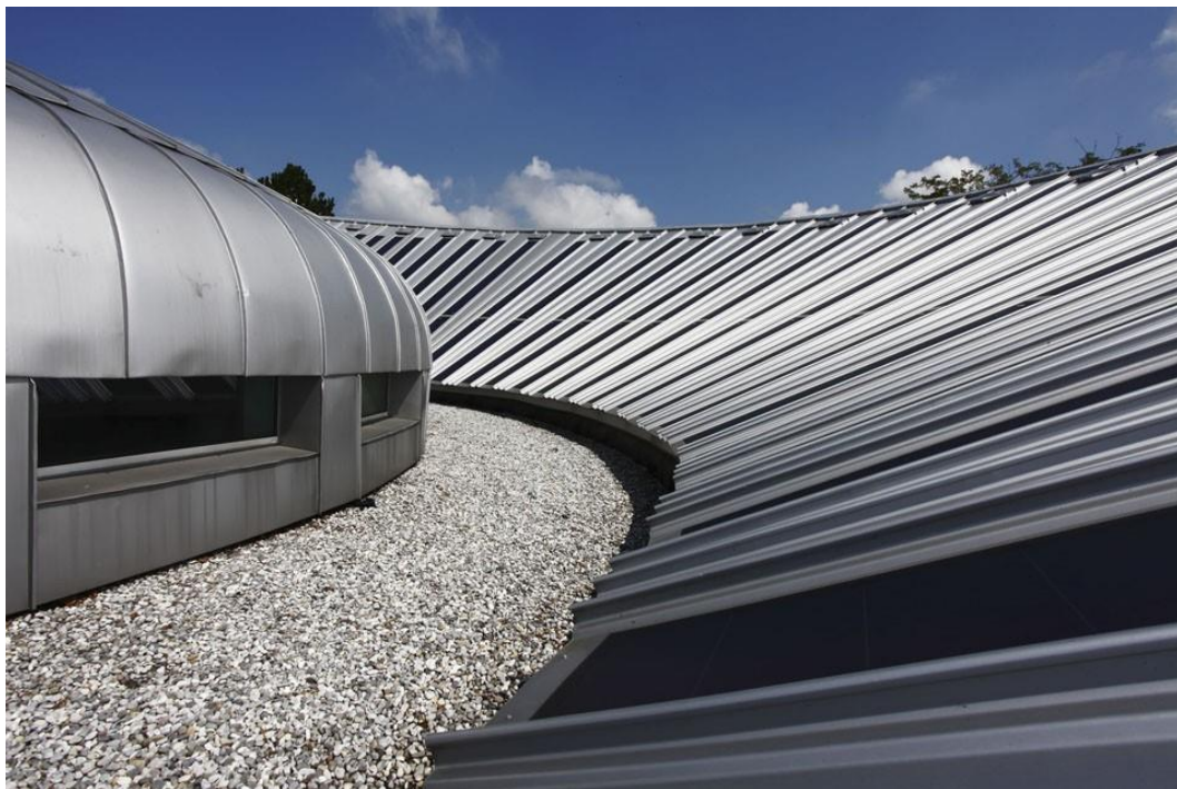
Figure 2.14. The image of Pitched roof in Folzano Kindergarten (Source: URL 8).
