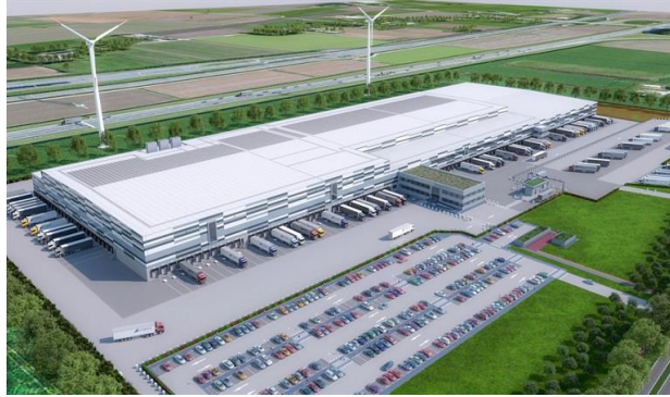
Şekil 4.5. Lidl Distribution Centre, Oosterhout. (Park15 Logistics, 2018)
