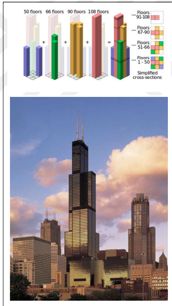
Şekil 2.6: Sears Tower (Willis Kulesi 2009).
