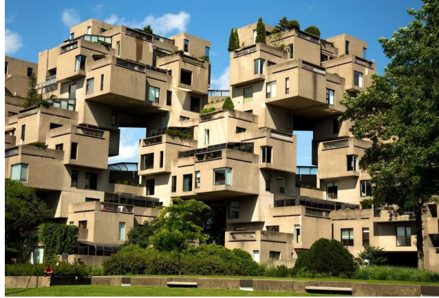
Şekil 4. 87 : Habitat '67, Cephede Brüt Beton Kullanımı, Moshe Safdie, Kanada. ( https://building.ca/more-than-half-century-after-construction-montreals-habitat-67-still-captivates/ )
