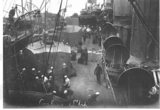
Figure 5.6: Coaling H.M.S. Natal c.1915. Note the marines pushing trolleys full of coal to the bunkers. NMM, C7137/R.
