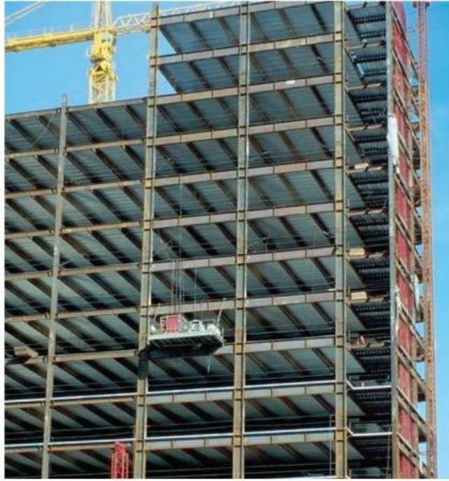
Figure 2.2 High rise steel moment frame structure under construction (FEMA P-749, 2010)
