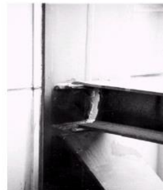
Figure 2.12 Damage to nonductile braces in the Kobe earthquake: fracture of welded links and web tear-out (left) and fracture of welded links (right) (Naeim, 2001)
