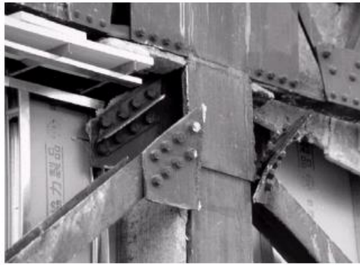
Figure 2.12 Damage to nonductile braces in the Kobe earthquake: fracture of welded links and web tear-out (left) and fracture of welded links (right) (Naeim, 2001)
