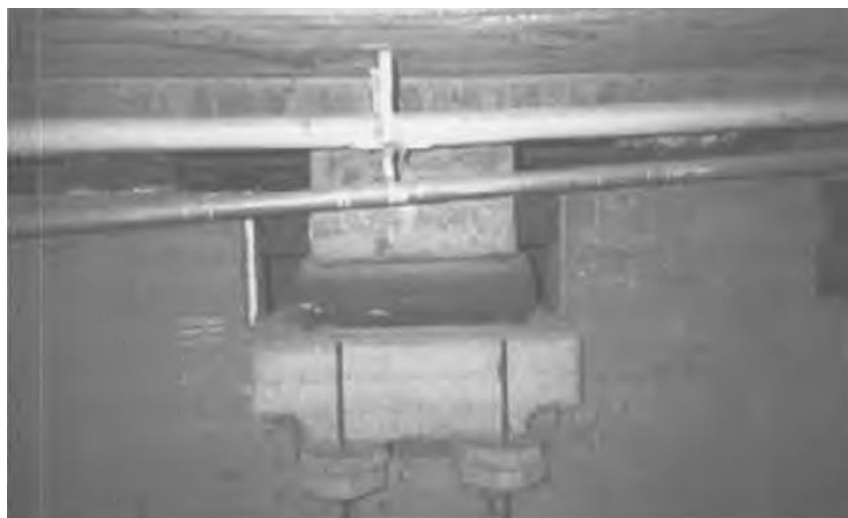
Figure 2.10 Bearings used in the Pestalozzi school (Kelly, 1981)
