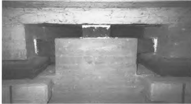
Figure 2.11 Seismic fuzes used in the Pestalozzi school (Kelly, 1981)
