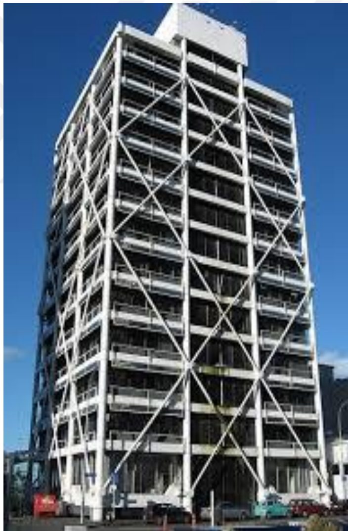
Figure 2.19 Union House, New Zealand (Boardman et al., 1983)
