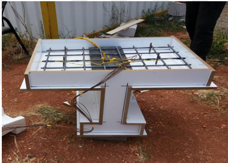
Figure 3.18 The I-Beam specimen before casting.
