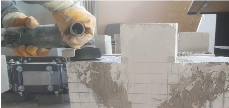
Figure 3.9 Adjusting the faces of the corbel by grinding machine
