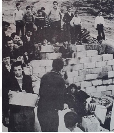
Figure 3.3 Construction of a gecekondu . 80 The making phase “suggests” heterogeneous concrete labour required for the collective task. Source: Tansı Şenyapılı, “Gecekondu Kadınının İşlevi,” Dünya , October 30, 1978.
