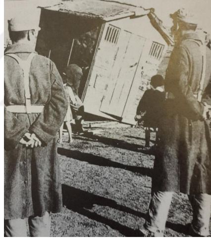
Figure 1.3 Demolition of a gecekondu .
