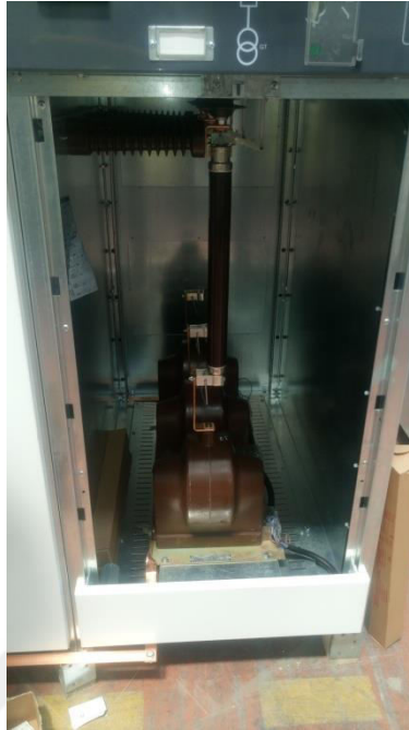
Figure 1-1 A gas insulated MV voltage transformer installed in a 36kV 630A switchgear equipment
