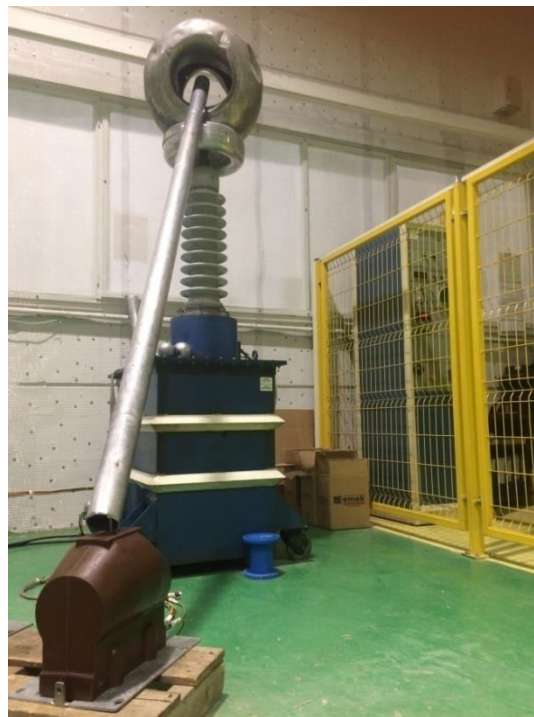
Figure 5-4 Partial discharge test setup
