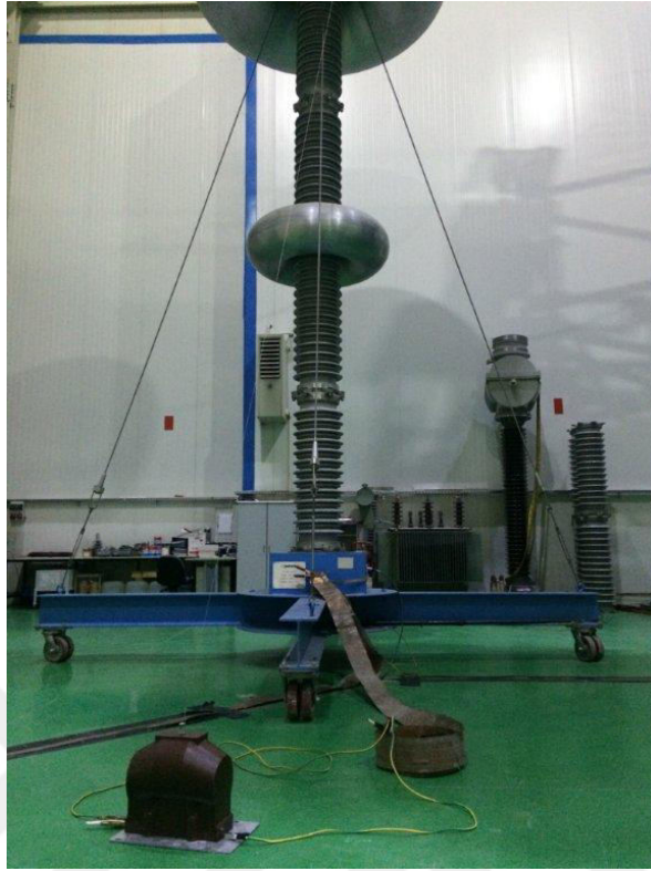
Figure 5-1 Standard lightning impulse test setup
